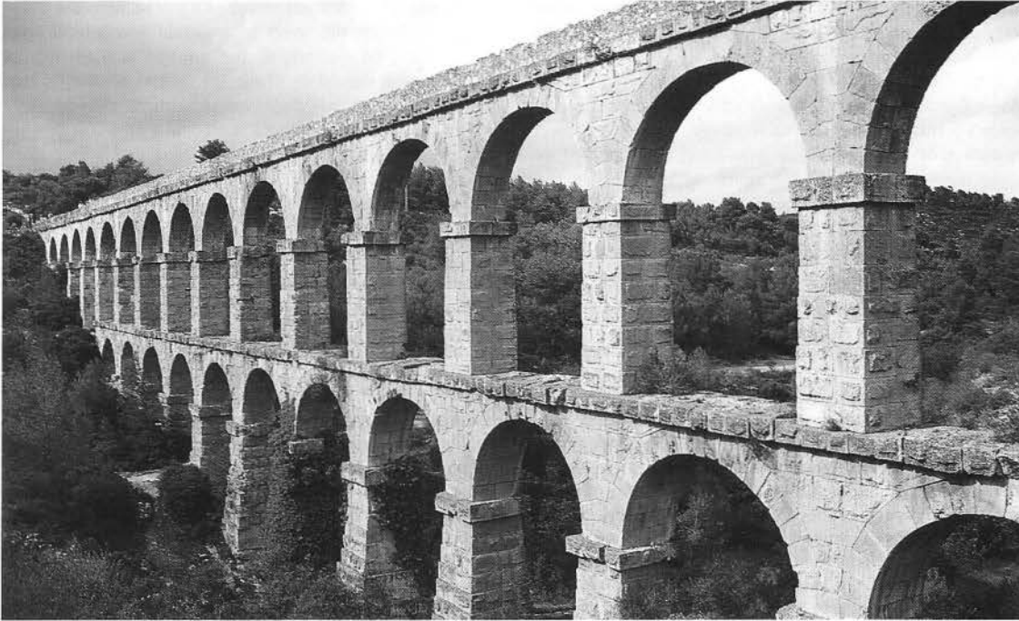
Roman Aqueduct Near Tarragona, Spain How to provide an adequate supply of water was a problem posed by the growth of Roman towns and cities. Aqueducts channeled water from a source, sometimes many miles away, to an urban complex, using only the force of gravity. To bring an aqueduct from high ground into the city, Roman engineers designed long, continuous rows of arches that maintained a steady downhill slope. Roman troops were often used in such large-scale construction projects. Scholars sometimes can roughly estimate the population of an ancient city by calculating the amount of water that was available to it. (Rober: Frerck/Woodfin Camp & Associates)
