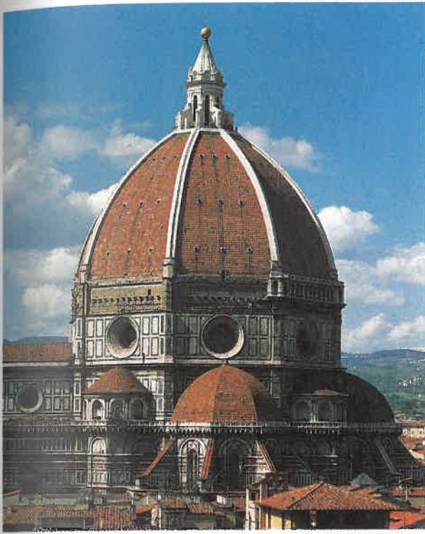
FIGURE 10.9 Florence Cathedral, 1420–1436 Brunelleschi's dome for the Cathedral of Florence was an architectural wonder. The architect creatively used ribs to support the dome's weight.
